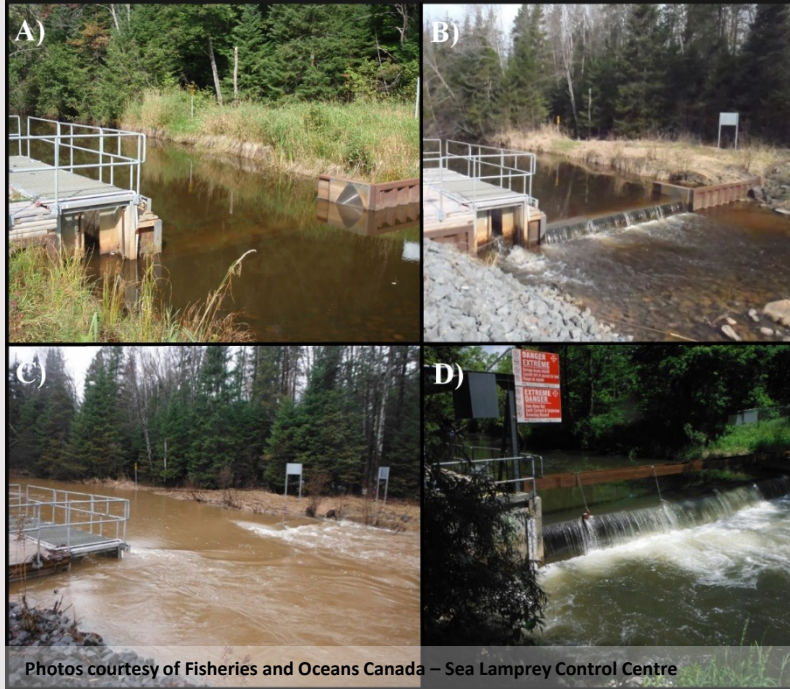
Big Carp River, Lake Superior, ON, inflatable crest barrier operating with (A) barrier down, (B) barrier up, (C) barrier up during flooding, and (D) Big Creek, Lake Erie, ON, barrier with beam used to lift the crest when the control system failed.
