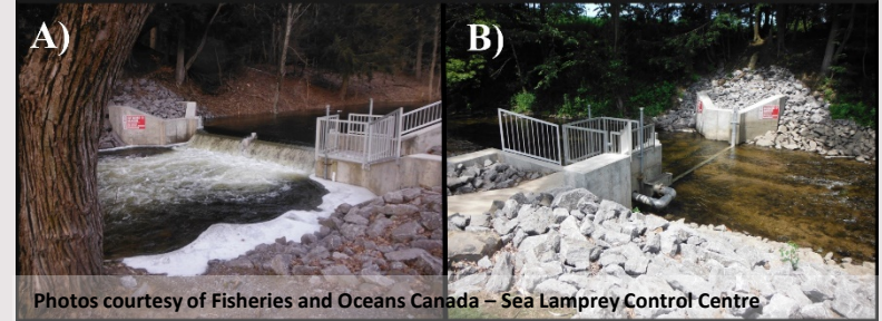
Seasonal barrier on Orwell Creek, Lake Ontario, NY with (A) stoplogs in and (B) stoplogs out during sea lamprey migration.
