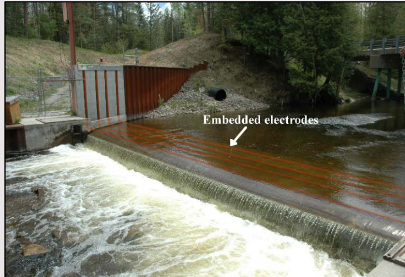
The combined graduated field fish barrier (GFFB) and fixed-crest barrier on the Ocqueoc River, Lake Huron, MI. Note the electrodes mounted along the barrier crest and vertical side walls. Photo courtesy of the Great Lakes Fishery Commission.
